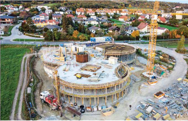
The construction of the new R&D center in Großhöflein is in full swing.
