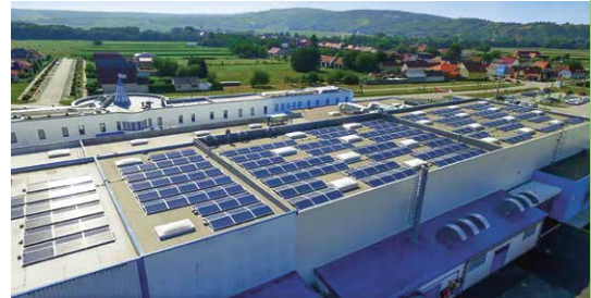
Photovoltaic system in Vaskeresztes
